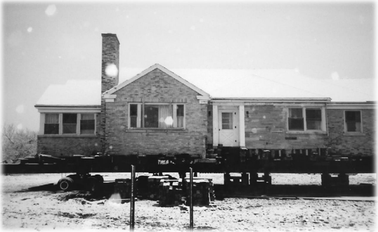
Figure 1: Structure placed on a wheeled vehicle for relocation to a new site
